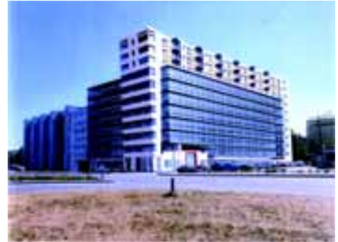
Admiral's House – Merko bets companies will buy their new office space, not rent.
