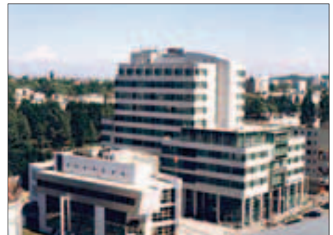
Baltic Business Centre (14 000 sqm) is a modern office building in Gdynia
