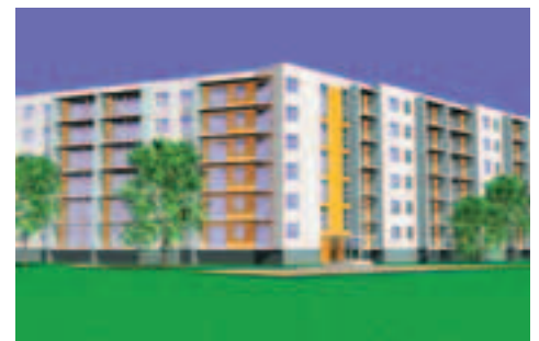
Dzimtā sēta – 72 apartment building in Purvciems suburb, Riga. Completion in second half of 2005.
