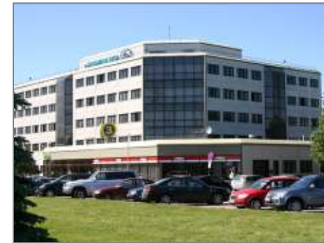
TV3 Building 28 000 sqm Office / Factory Tallinn
